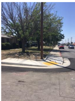
Curb cut constructed at Bernard/Magnolia Bus Stop
