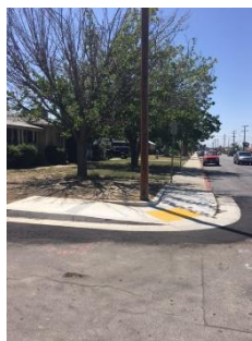
Curb cut constructed at Bernard/Magnolia Bus Stop
